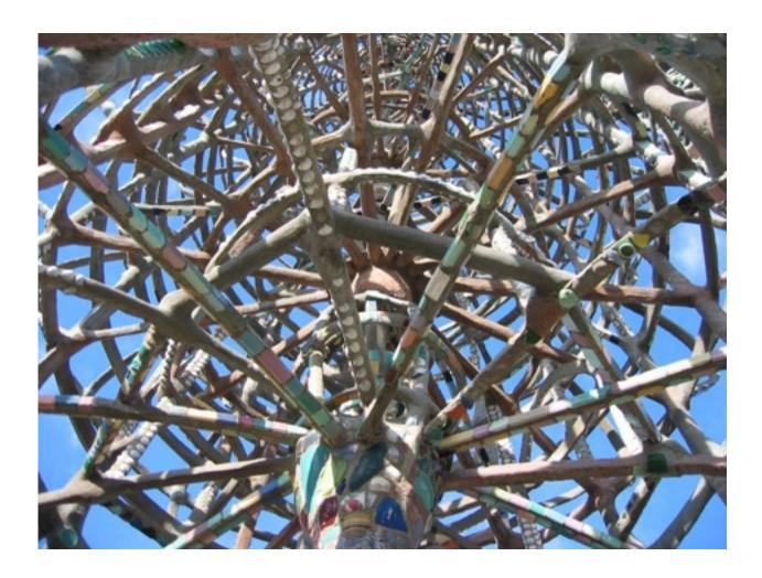
The withstanding of weather and moisture for over half a century have caused pieces of tile and glass to become loose on the towers, which are conserved for reattachment in the ongoing restoration work. The structures suffered little from the 1994 Northridge earthquake in the region, with only a few pieces shaken loose.
